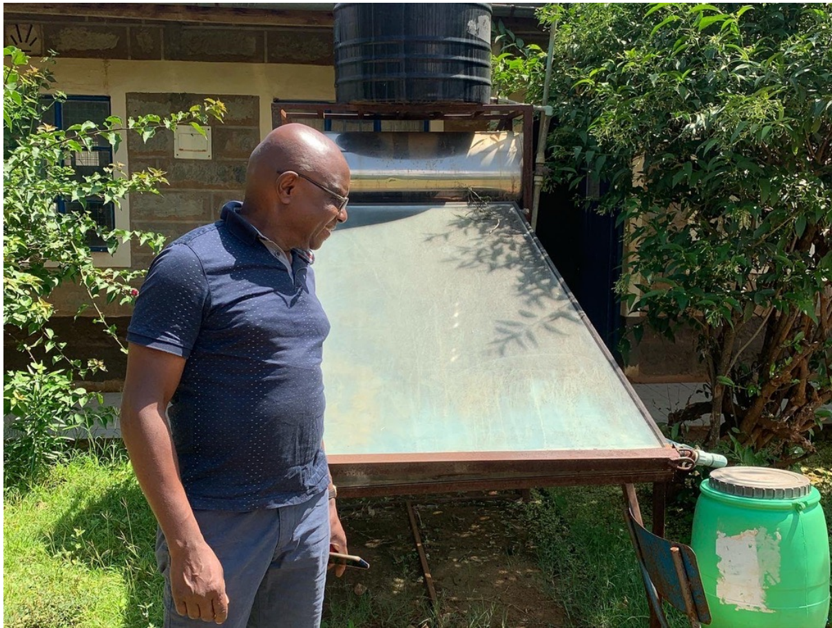
John inspecting the hot water system at Betty's Academy
